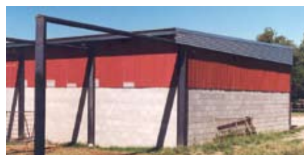
Bunker with flat sliding roof
