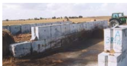
Concrete block bunkers
