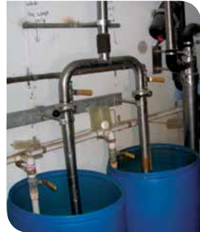
Figure 8 Wash manifold (example only). Cleaning solution uptake is manually controlled by using the lever valves.
