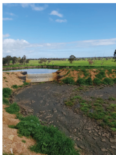
The upgraded effluent management system at White Rocks
