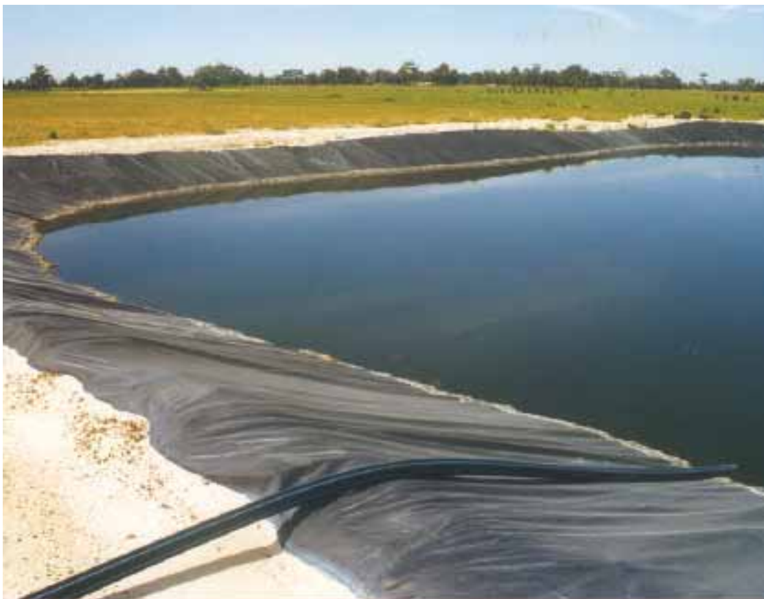
Plastic-lined effluent ponds are an expensive option for permeable soils
