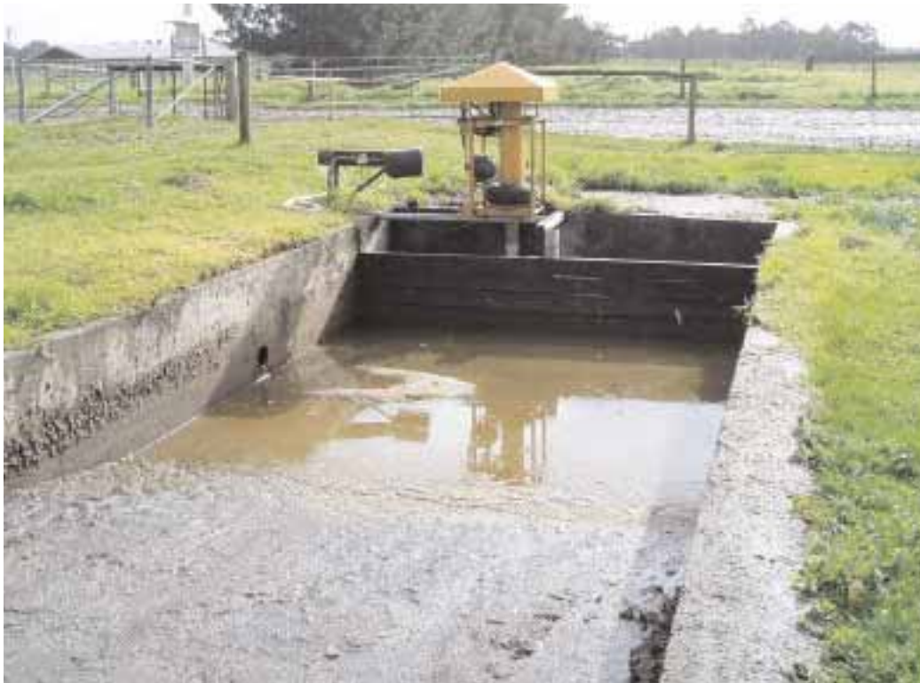
Trafficable sump with Rankin pump at the Vasse Research Centre, Busselton
