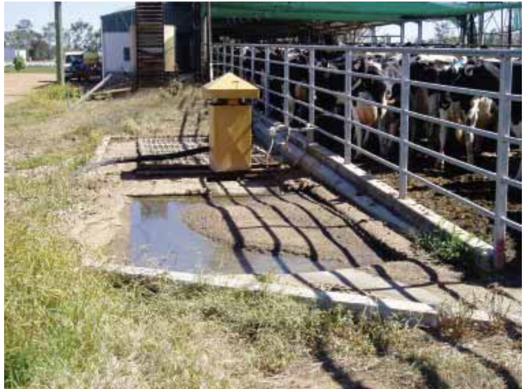
Sump conveniently located along side the yard at the Hanks dairy in Harvey
