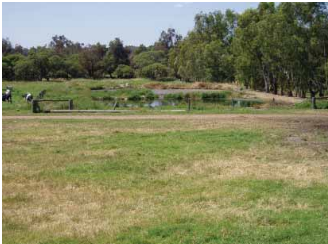
FIGURE 6.7. Two pond system at Hayes Dairy in Cookernup
