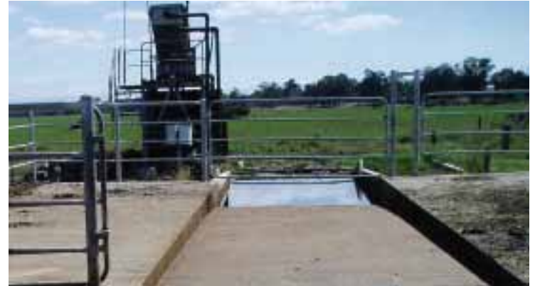
Wash down water is channelled into the effluent bunker at the Bell Dairy
