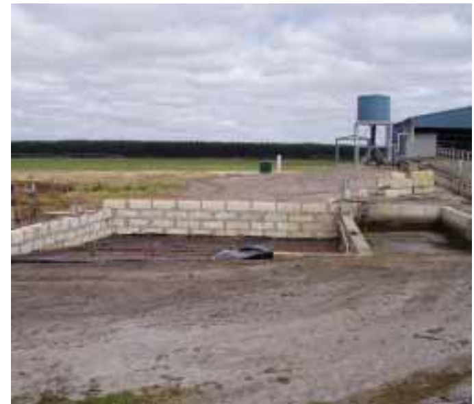
FIGURE 6.2. Diagram of a solids removal trench with a floating scum barrier made of polyethylene pipe
