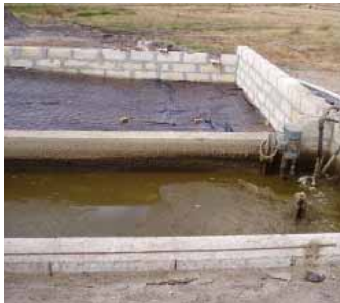
FIGURE 6.3. Drainage wall constructed of reconstituted limestone blocks
