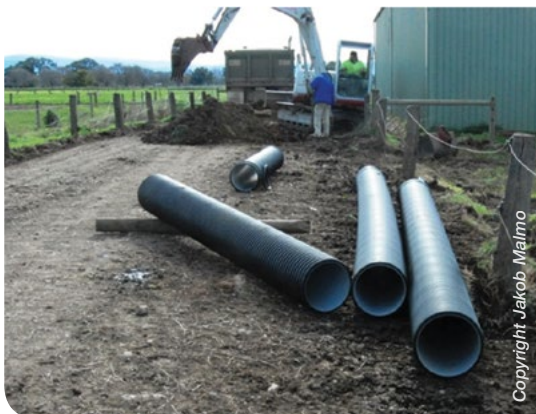
These photos illustrate construction of a culvert to drain water under laneway
