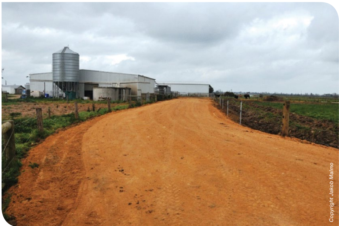
Drainage ditch on the paddock side of laneway fence
