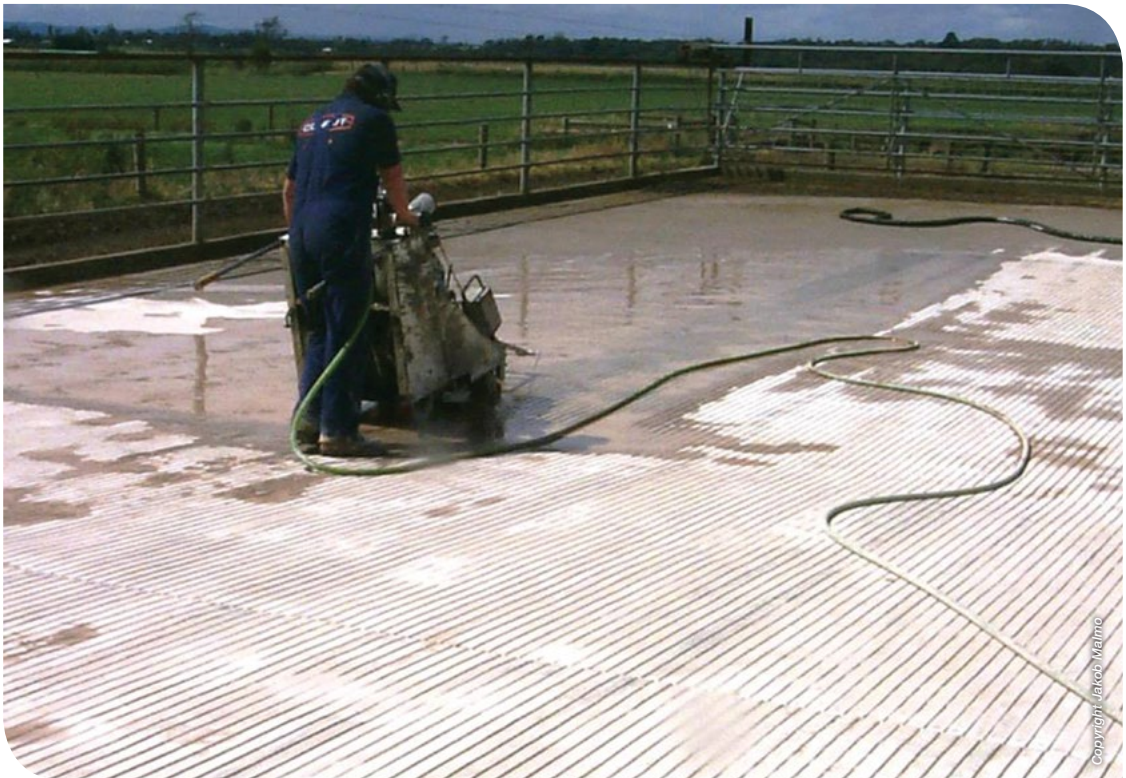
Grooving the yard in the direction of cow flow
