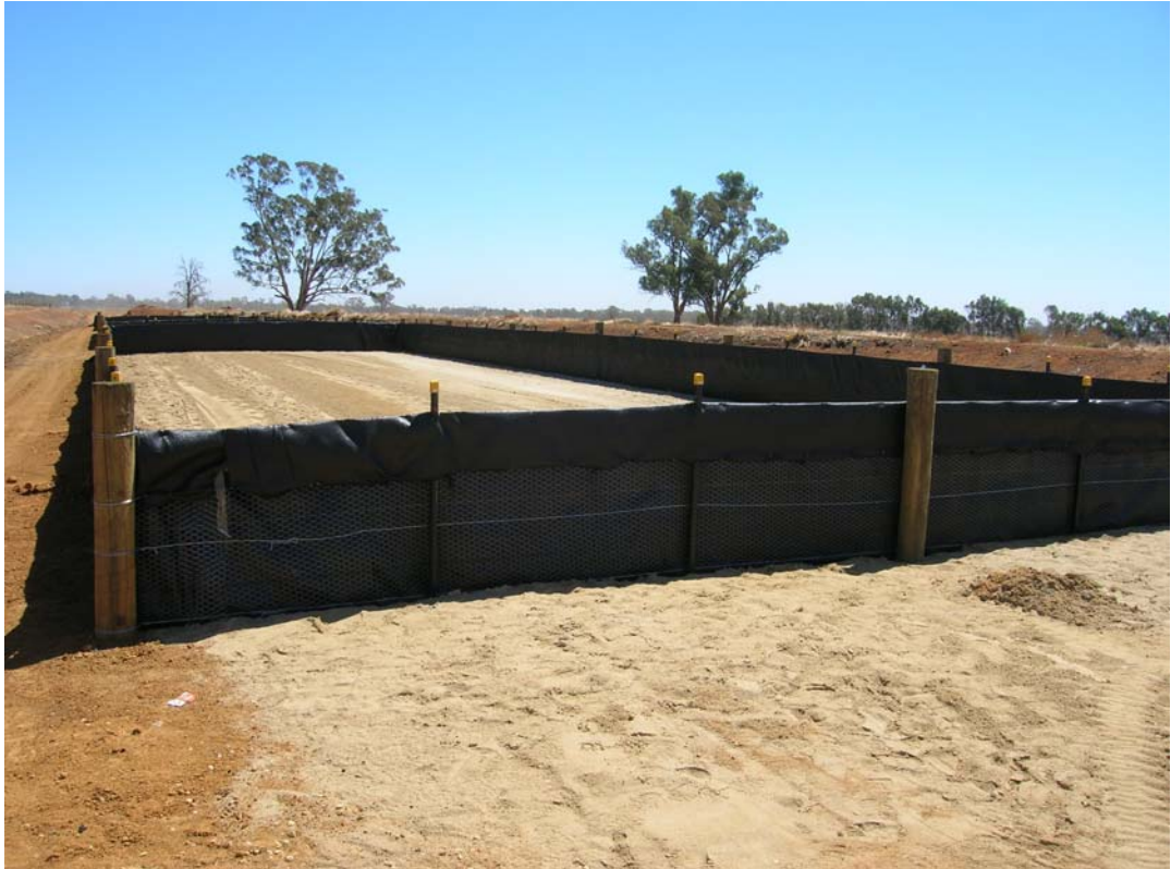
Figure 1. Empty drying bay with shadecloth fence (photo courtesy of Australian Pork Limited & QAF Meats).
