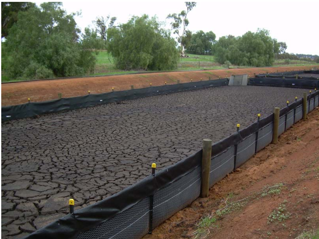
Figure 2. Drying bay before clean-out (photo courtesy of Australian Pork Limited & QAF Meats).
