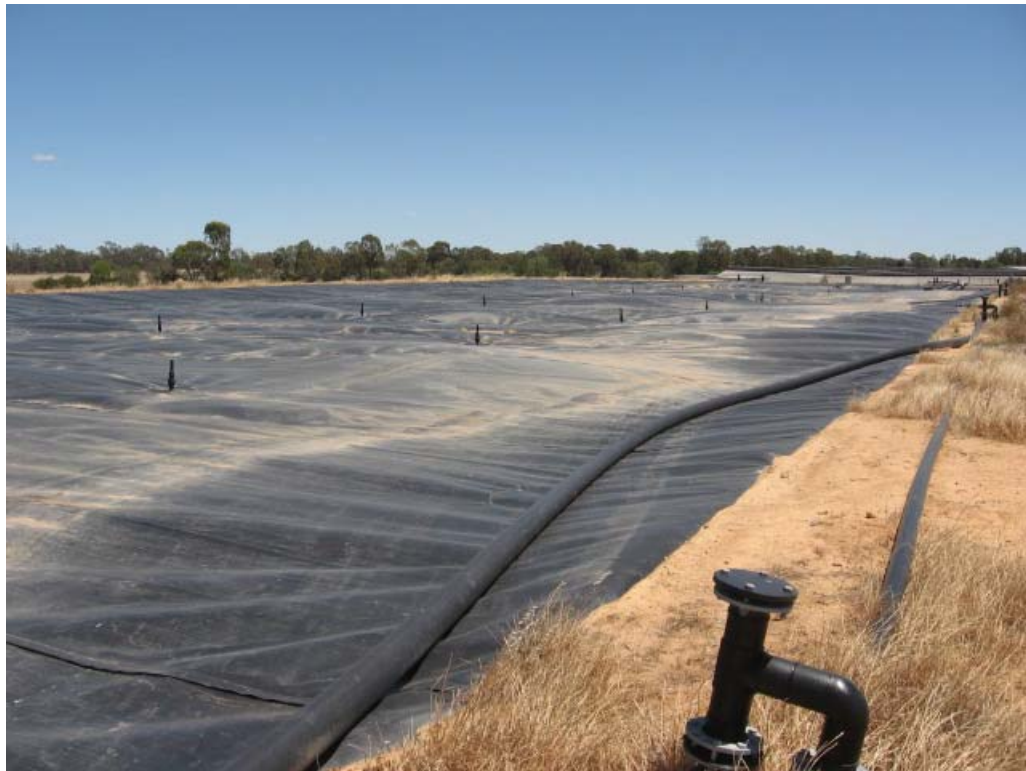
Figure 2. Enhanced covered anaerobic pond (photo courtesy of George Western Foods).
