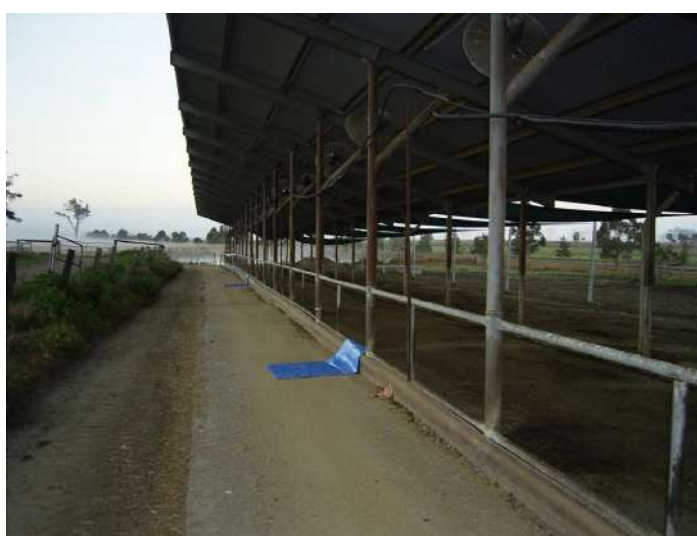
Figure D. Placing the tarpaulins before feed-out (one sided trough)
