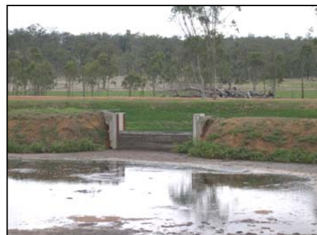
Settling basin with drop board weir
