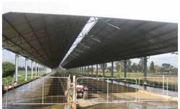
Fully concreted feedpad with nib wall, central feed alley, solid roof and flood wash system
