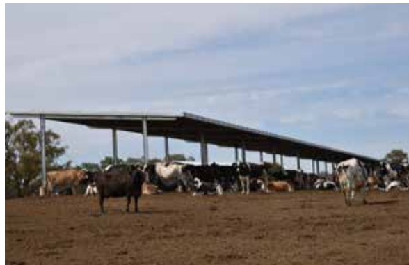
Figure 16. Centralised shade shelters at a dairy dry lot with a north-south orientation
