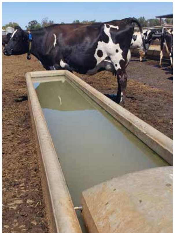
Water trough with concrete drinking apron to prevent runoff onto earthen pen and pugging damage around the trough
