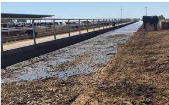
Flood washing of concrete cow feeding alleyways
