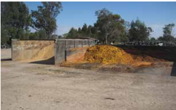
Concrete bunkers for storing by-products
