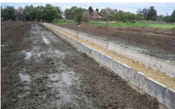
PMR fed out with mixer wagon into 2 types of modular concrete troughs (3-sided profile and 'J' profile). On trough with J profile, note strip of timber added to low side
