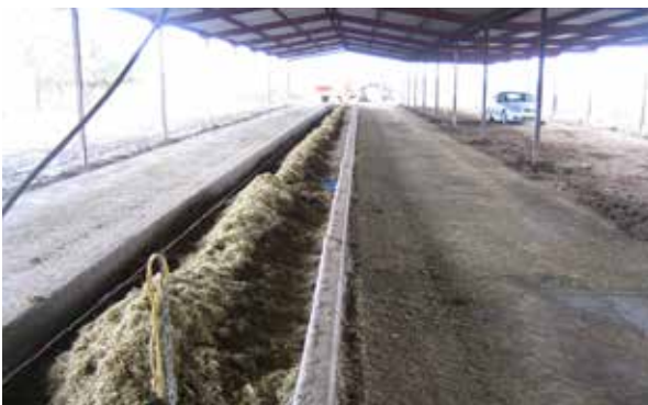
Wider square-profiled trough on earthen pad under solid roof
