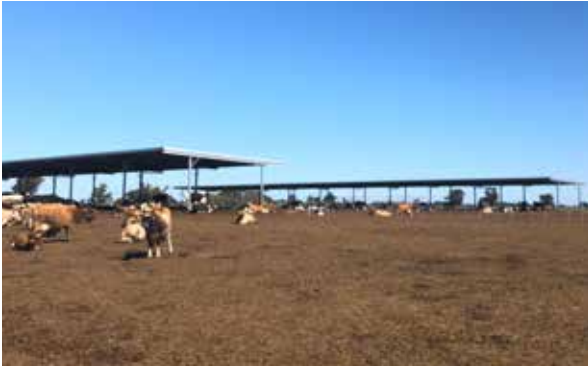
Shade shelters at a dairy dry lot with a north-south orientation
