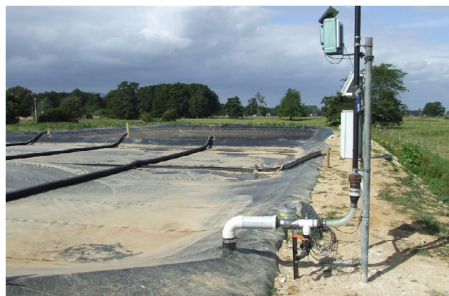
Covered anaerobic pond and candlestick flare. Photo courtesy of NIWA
