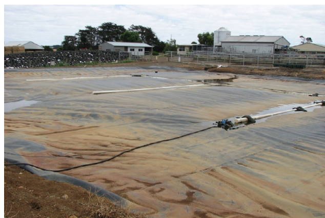
Covered anaerobic pond. Photo courtesy of DemoDAIRY
