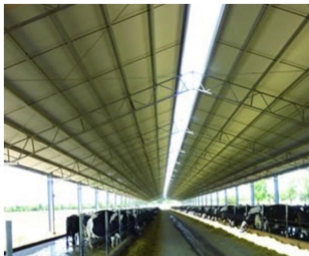
This roof slope is 18° with a 500mm vent at the apex. Eaves are 4.3 m high, and 6.9m at apex. The shed runs north-south with 3% slope on patterned cement floor. Feed troughs are 1.2m wide inside, 400mm high and 100mm thick.
