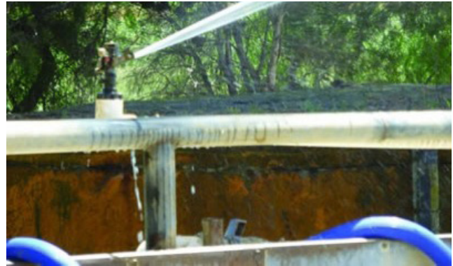
The sprinklers generate a semi-circle spray pattern that is directed towards the yard side of the shed
