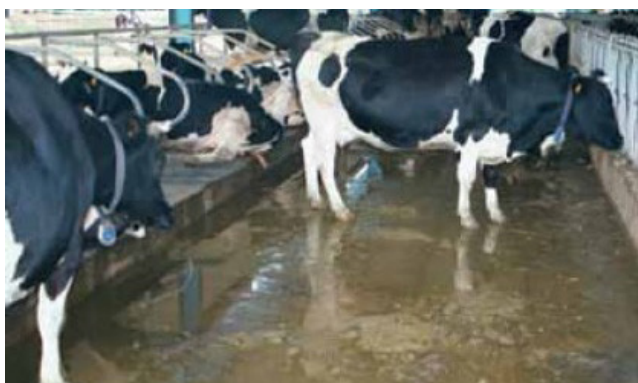
Note the poor drainage due to the lack of slope. The freestall shed has fans and sprinklers but is not linked to good drainage – a recipe for high mastitis levels
