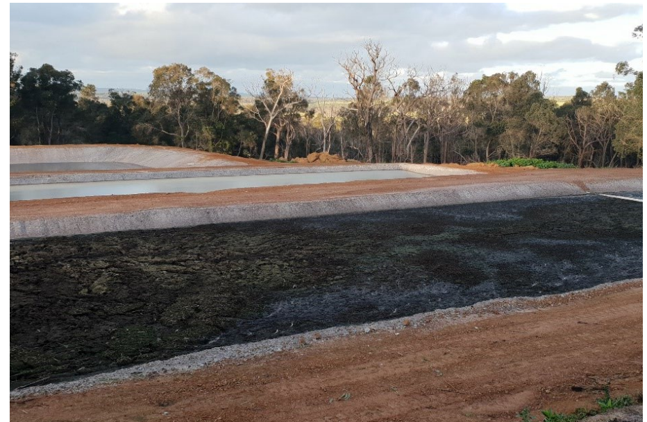
A primary solids pond is a low maintenance option to separate solids and liquids
